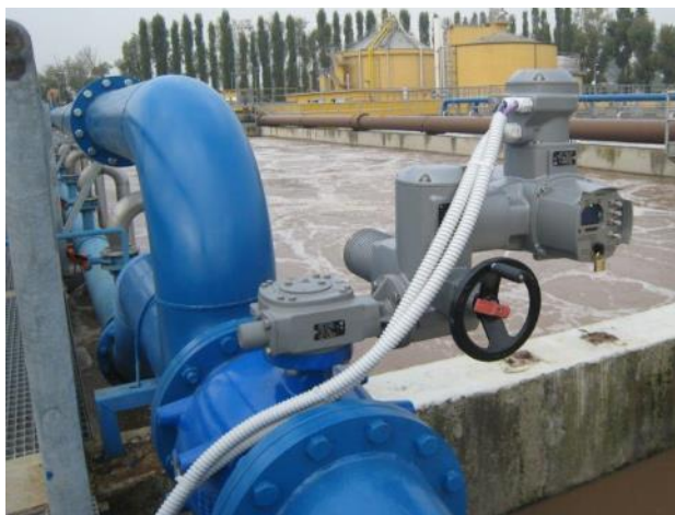
Figs. 1 & 2 — Plunger valve for regulating air flow into a nitrification tank: the valve is equipped with an electrical actuator.
