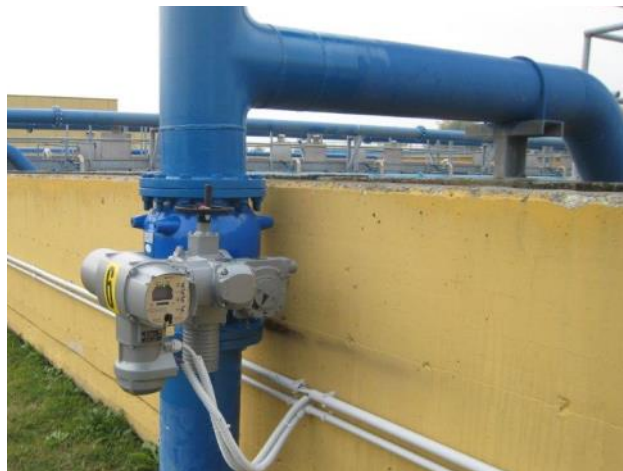
Figs. 1 & 2 — Plunger valve for regulating air flow into a nitrification tank: the valve is equipped with an electrical actuator.
